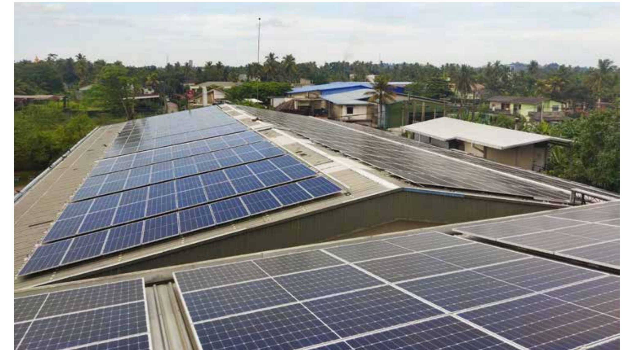
Solar panel installation – A&E Sri Lanka
